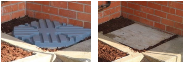
Figure 6: Concrete or heavy duty plastic slabs to be placed under the storage tank.
