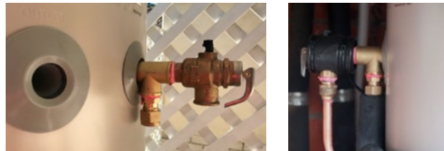
Figure 8: A tee connection for heat pump return line and PTRV valve (AP315AGLH model number only).
