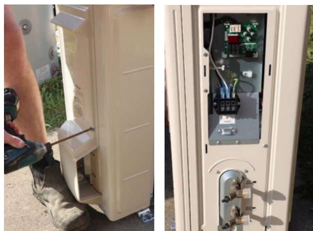
Figure 16: How to remove the piping cover from heat pump.
